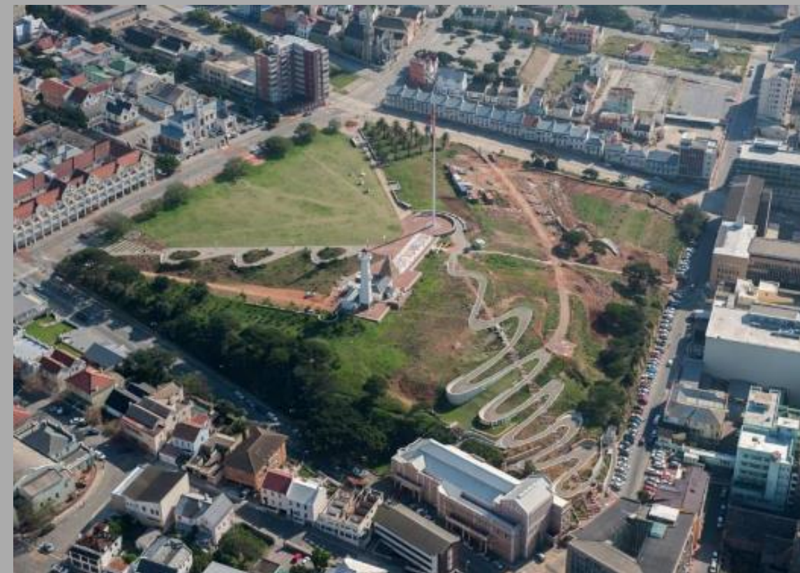
Aerial View of the Works Under Construction
