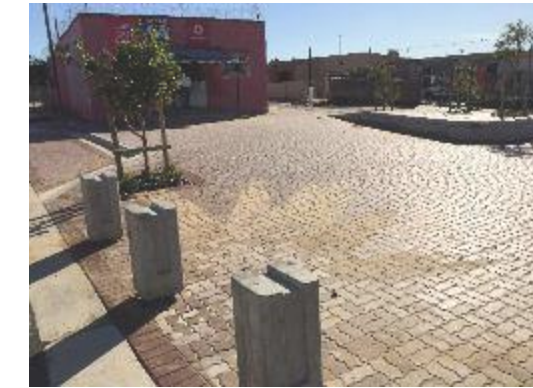
Zone 3A park construction.
