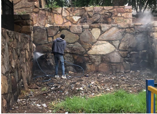
Chemical washing of graffiti was a challenge on the over 100 year-old stone walls- but succeeded!
