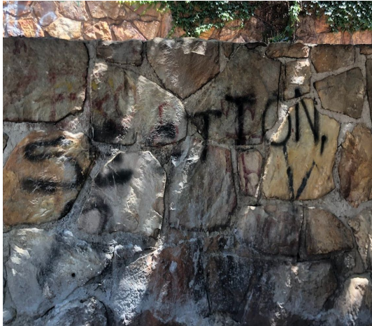
Chemical washing of graffiti was a challenge on the over 100 year-old stone walls- but succeeded!
