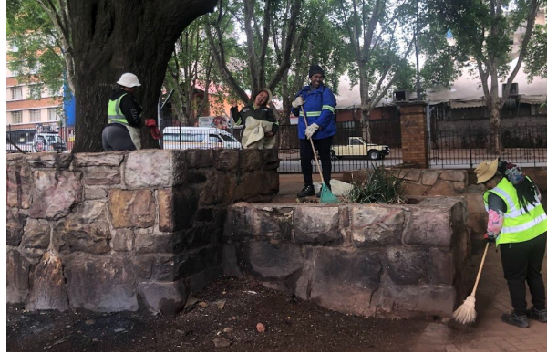
Chemical washing of graffiti was a challenge on the over 100 year-old stone walls- but succeeded!
