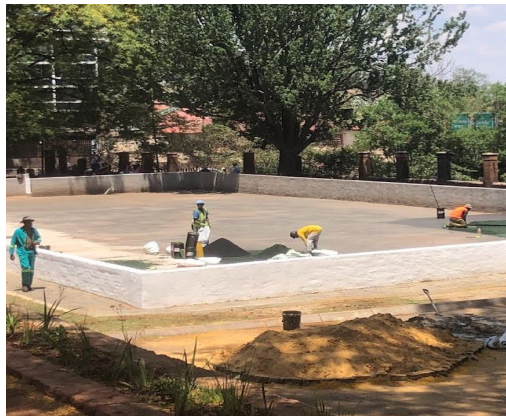
Rubberizing. Paving apron by JCP.
